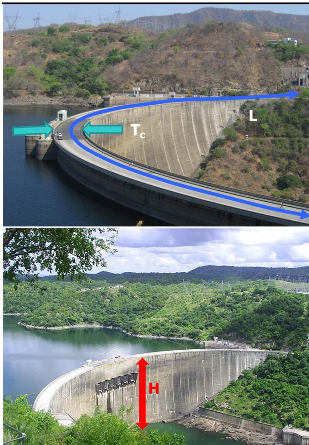
Figure 2.2 Dimensions of the Kariba Dam Wall
