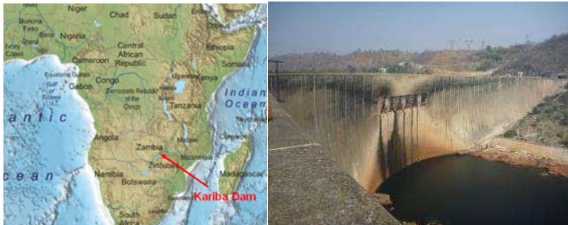
Figure 1 - The Kariba Dam General Location
