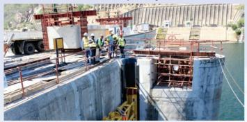
The Kariba Dam's six spillway gates, responsible for controlling water discharge, have faced operational challenges caused by Alkali Aggregate Reaction (AAR). This condition leads to swelling in the concrete, impeding smooth gate movement.
