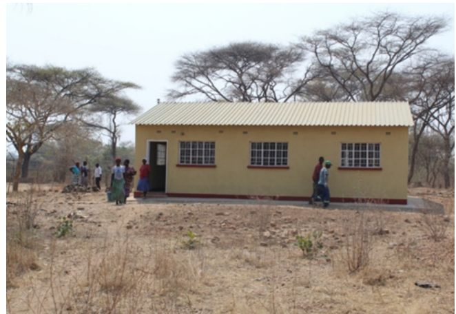
Figure 30. A staff house constructed at Simchembu Clinic
