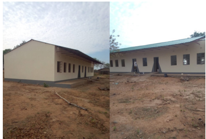
Figure 29. A 1x2 classroom block under construction at Ntivule Primary School
