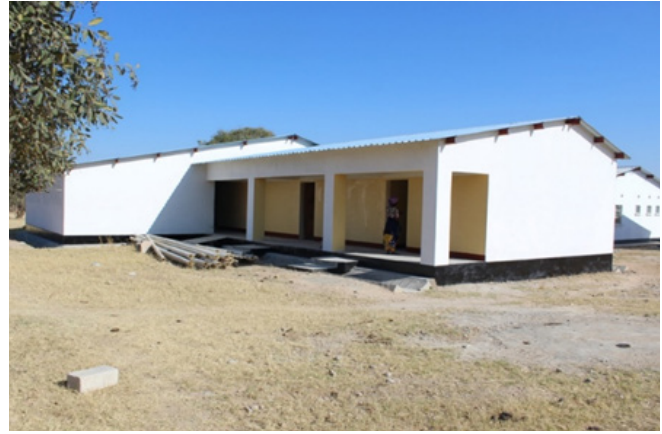
Figure 27. The OPD department under construction at Njabalombe clinic site
