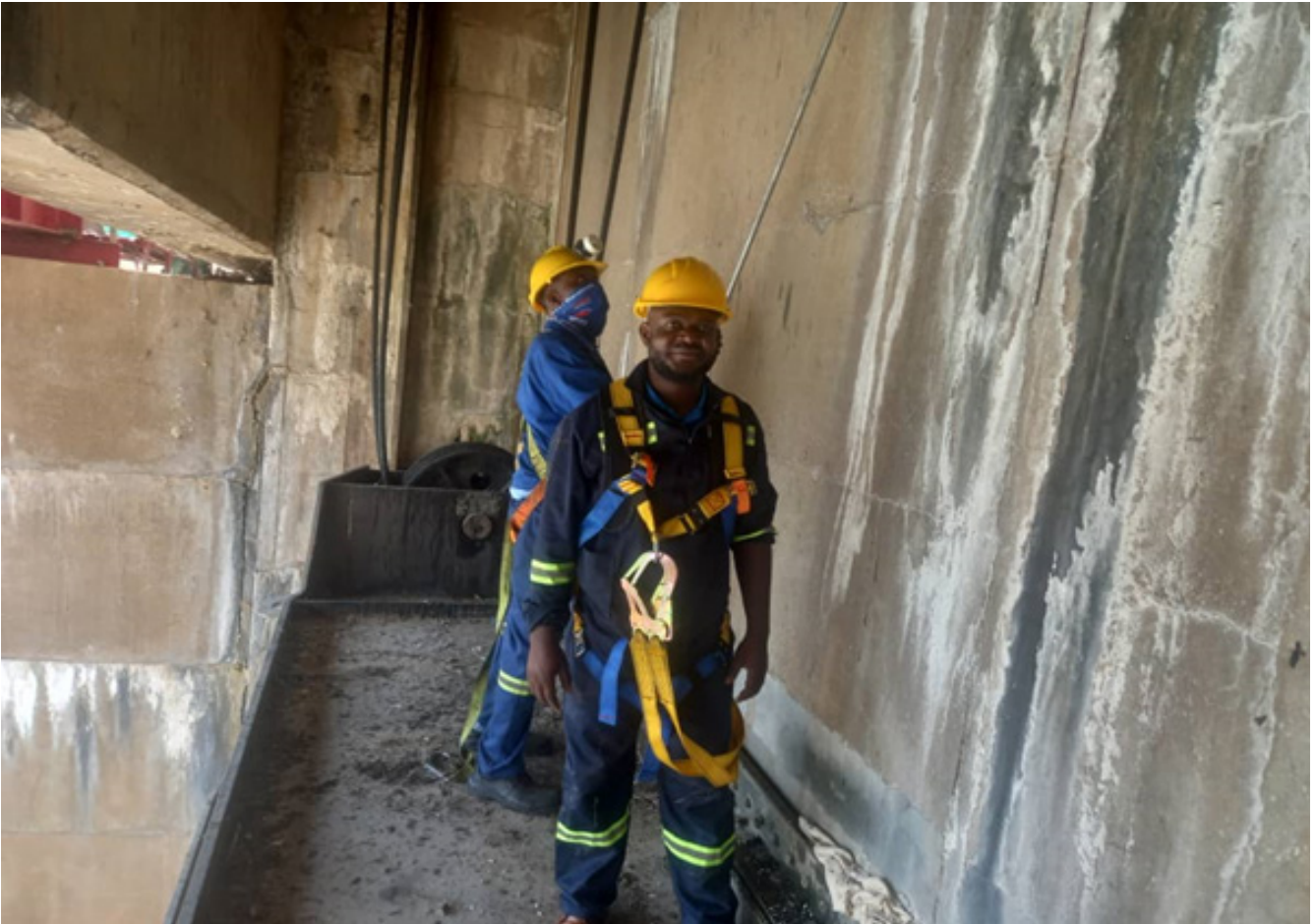
Figure 20. Maintenance works in preparation of raising floodgate no. 3.
