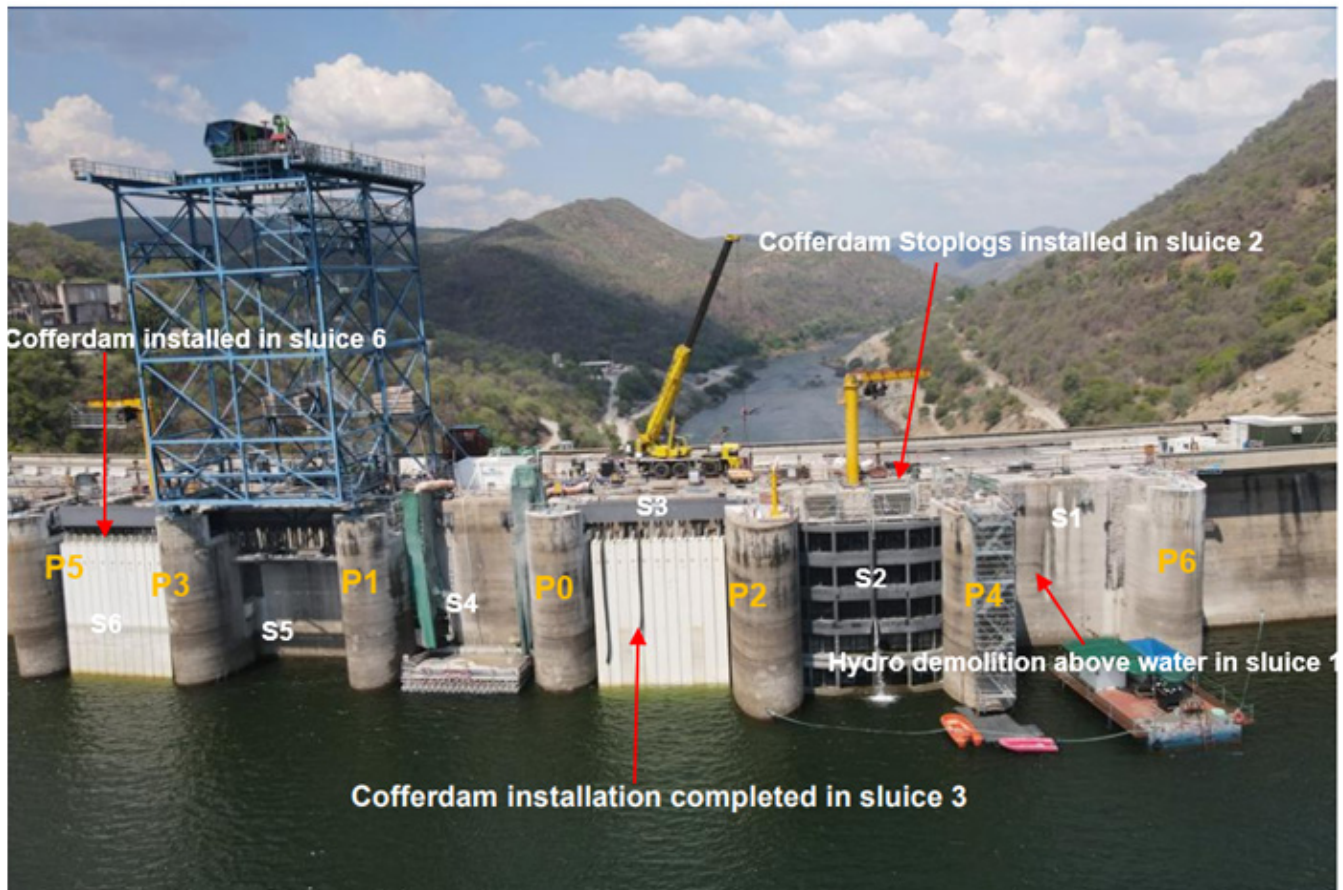
Figure 24. works at the spillway gates viewed from the upstream side (lake)
