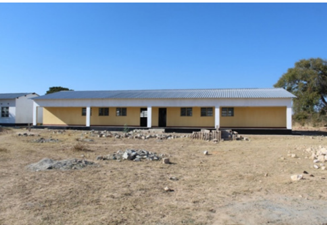
Figure 28. Admission ward under construction at Njabalombe Clinic site
