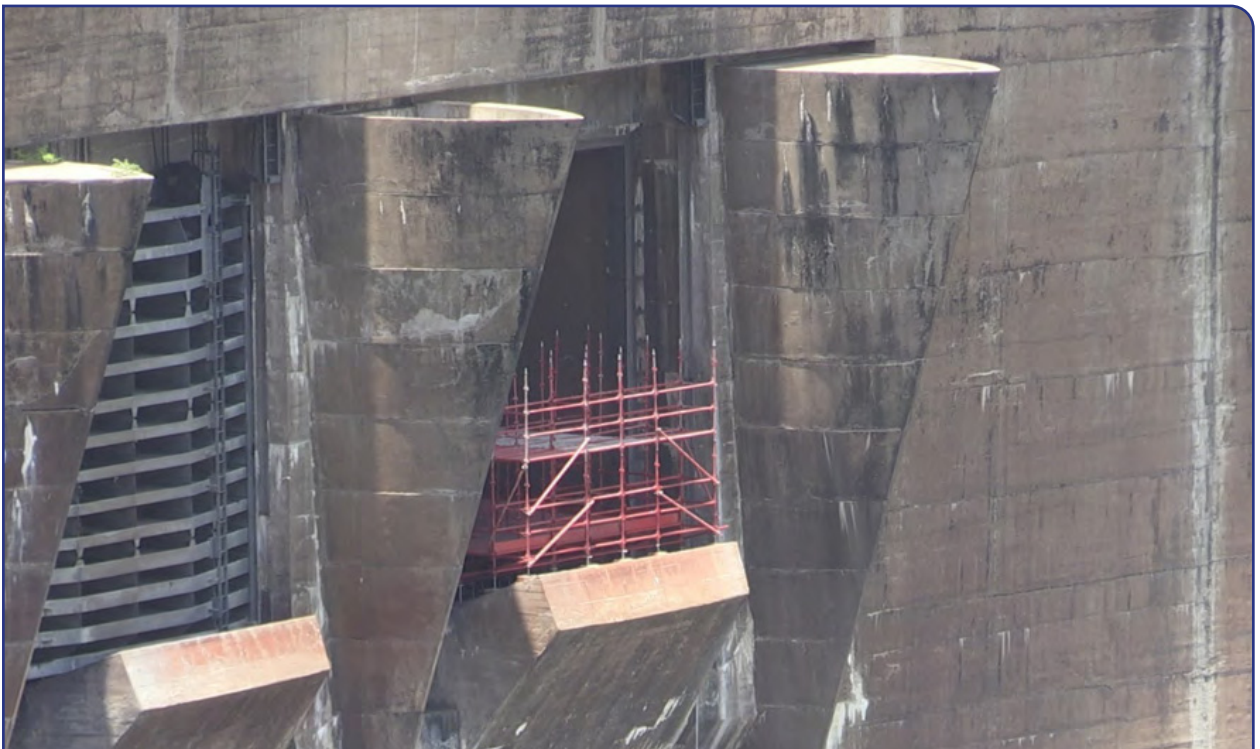
Downstream scaffold erection in Sluice 6 of the Spillway
