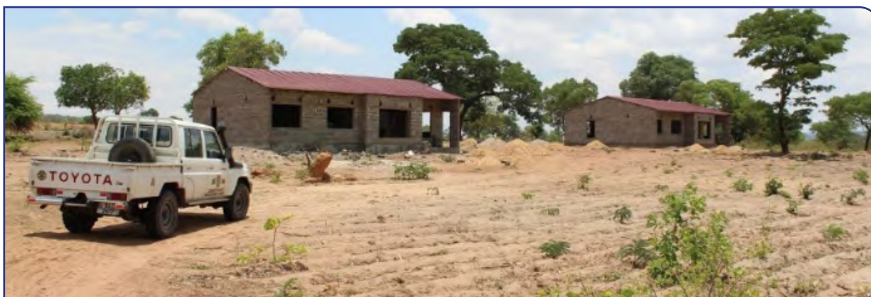
Construction of two staff houses at Nkandazovu Secondary School in Kalomo
