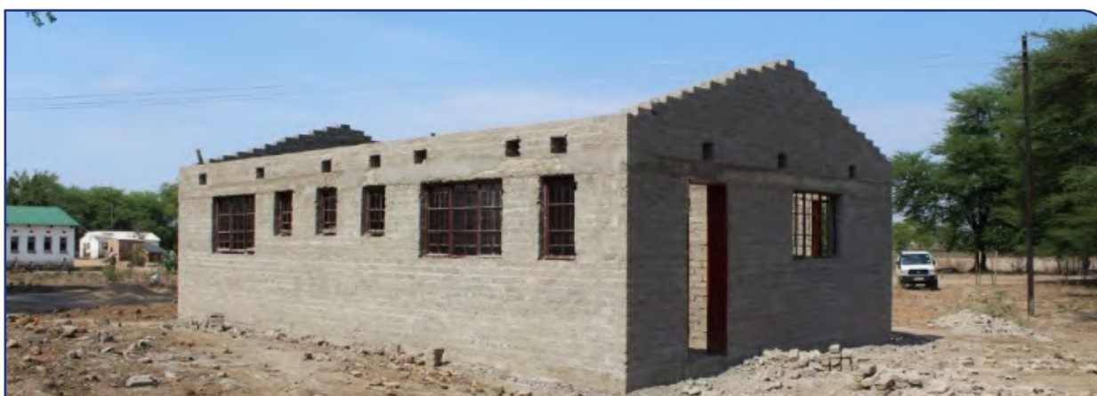
Construction of a staff house at Simchembu Clinic
