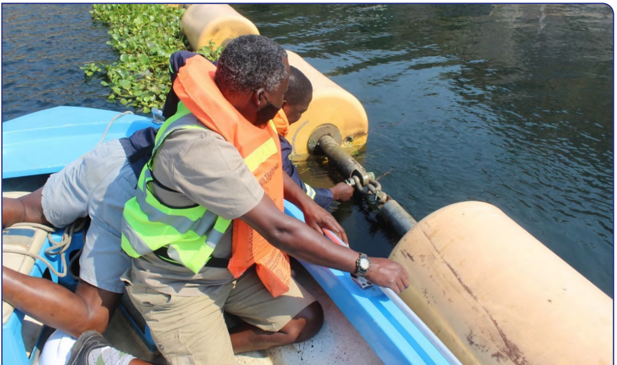
Hydrology team led by the Hydrologist Eng. Pherry Mwiinga inspecting the hyacinth traps just before the intake points
