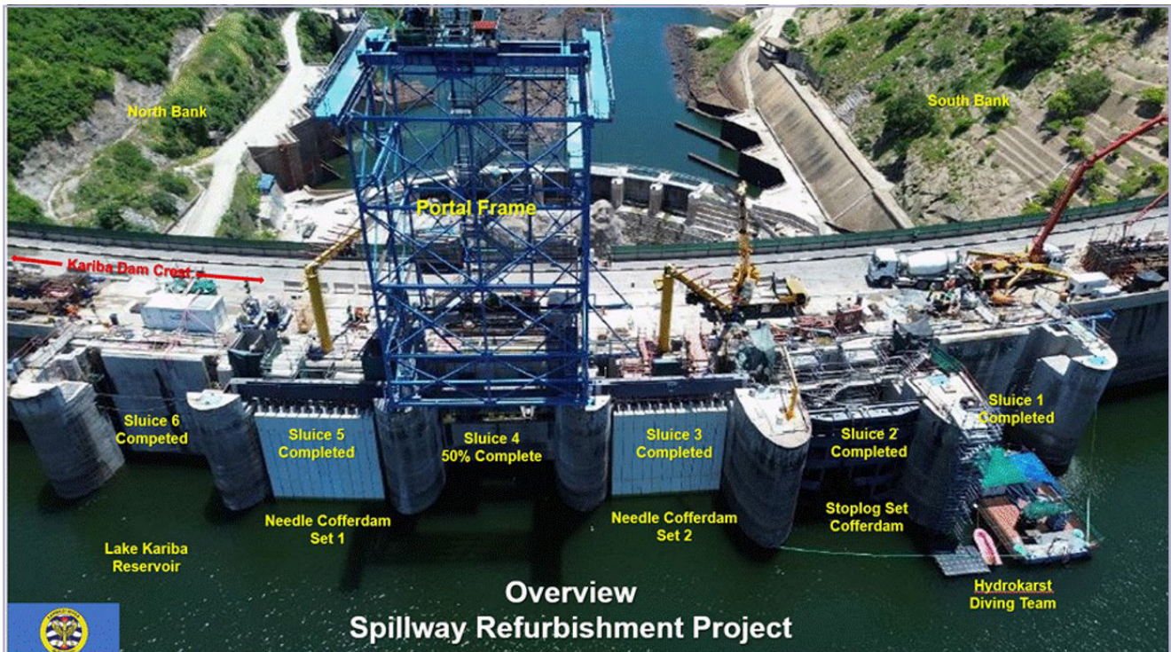
Figure: 33 Spillway refurbishment phase one works layout
