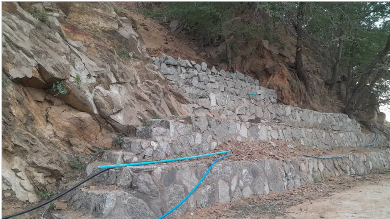
Figure 16: Phased construction and repair of the gulley at the hairpin bend.
