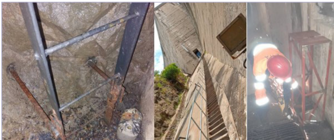
Figure 14: Installation of ladders (left), handrails (centre) and protecting instruments (right).
