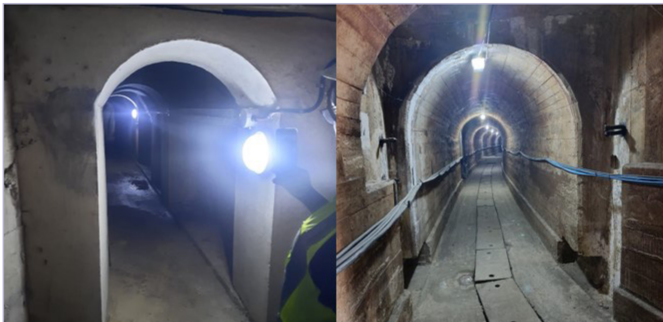
Figure 13: Extension of lighting in Adit A (left) and reduced spans in gallery A (right)
