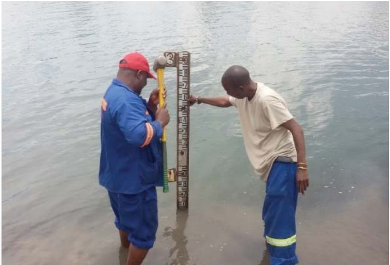
Fig. 40: Hydrology staff adjusting the 11-13m range gauge plate
