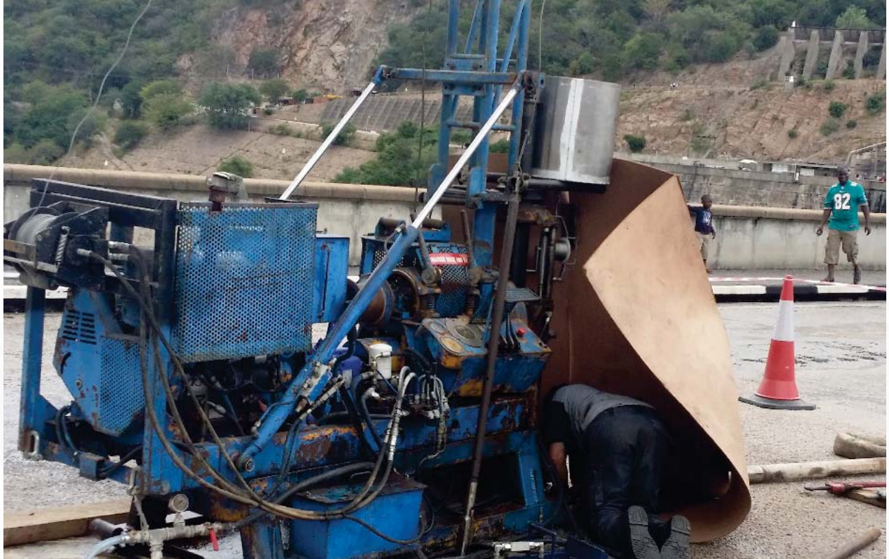
Fig. 9: Drilling rig at crest level
