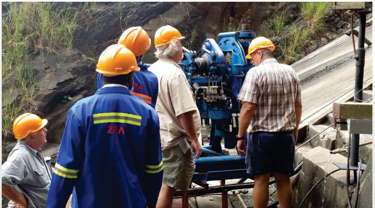
Fig. 10: Moving drilling rig into one of the dam galleries
