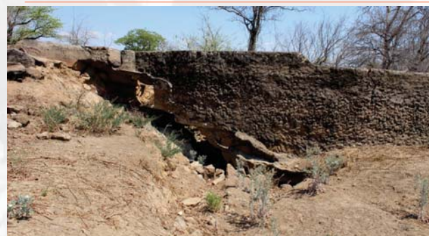
Fig. 18: Dam was cracked at the centre and undercut foundations on the left abutment
