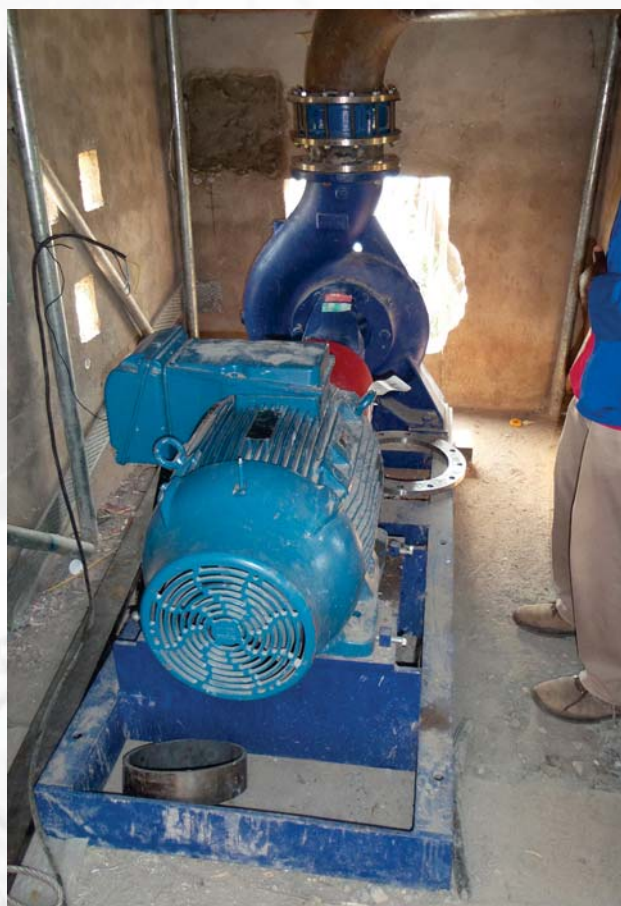
Fig. 20: New pump at Lusitu irrigation scheme
