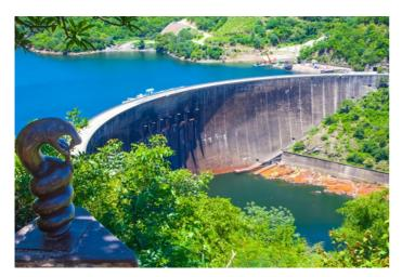
Management of the Kariba reservoir is mainly influenced by factors such as rainfall over the Zambezi Basin, inflows from the Zambezi River and its tributaries, outflows which include discharges through turbines, spillway gates and evaporation.
