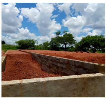
Figure 3: The foundation box for the 1x3 classroom block under construction at Nkandazovu Primary School
