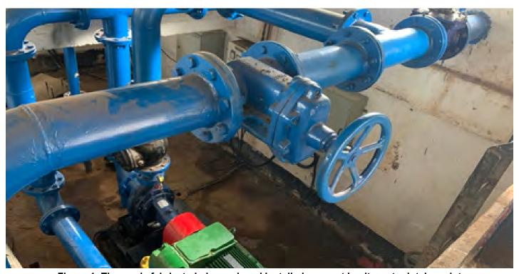
Figure 1: The newly fabricated pipework and installed pump at Lusitu water intake point Sinafala Secondary School, Gwembe District
